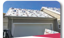
Roofing Inspections, installs, repairs, and replacements
