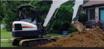
Traditional Messy Excavation Method
